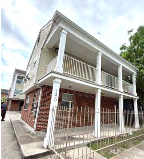
Front Building (Unit A) Front View
