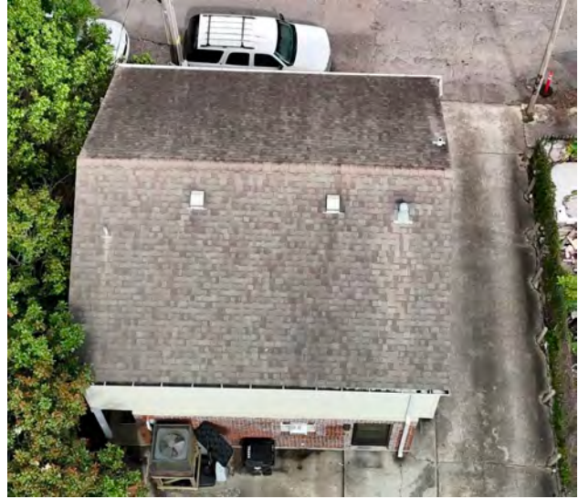
Front Building (Unit A) Aerial View
