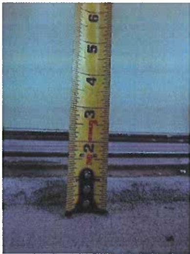
Threshold and change in level at primary entrance threshold exterior side, 1210 Rev. John Raphael Jr. Way.
