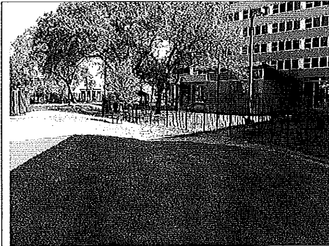
1. Area requiring drain.
